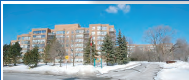
Cheerful 2 bedroom plus den, corner unit in Aurora's most popular condominium building. 24 hour security, Tons of natural light. Comfortable and spacious open concept living and dining room. Private underground parking. Asking $434,900.00
