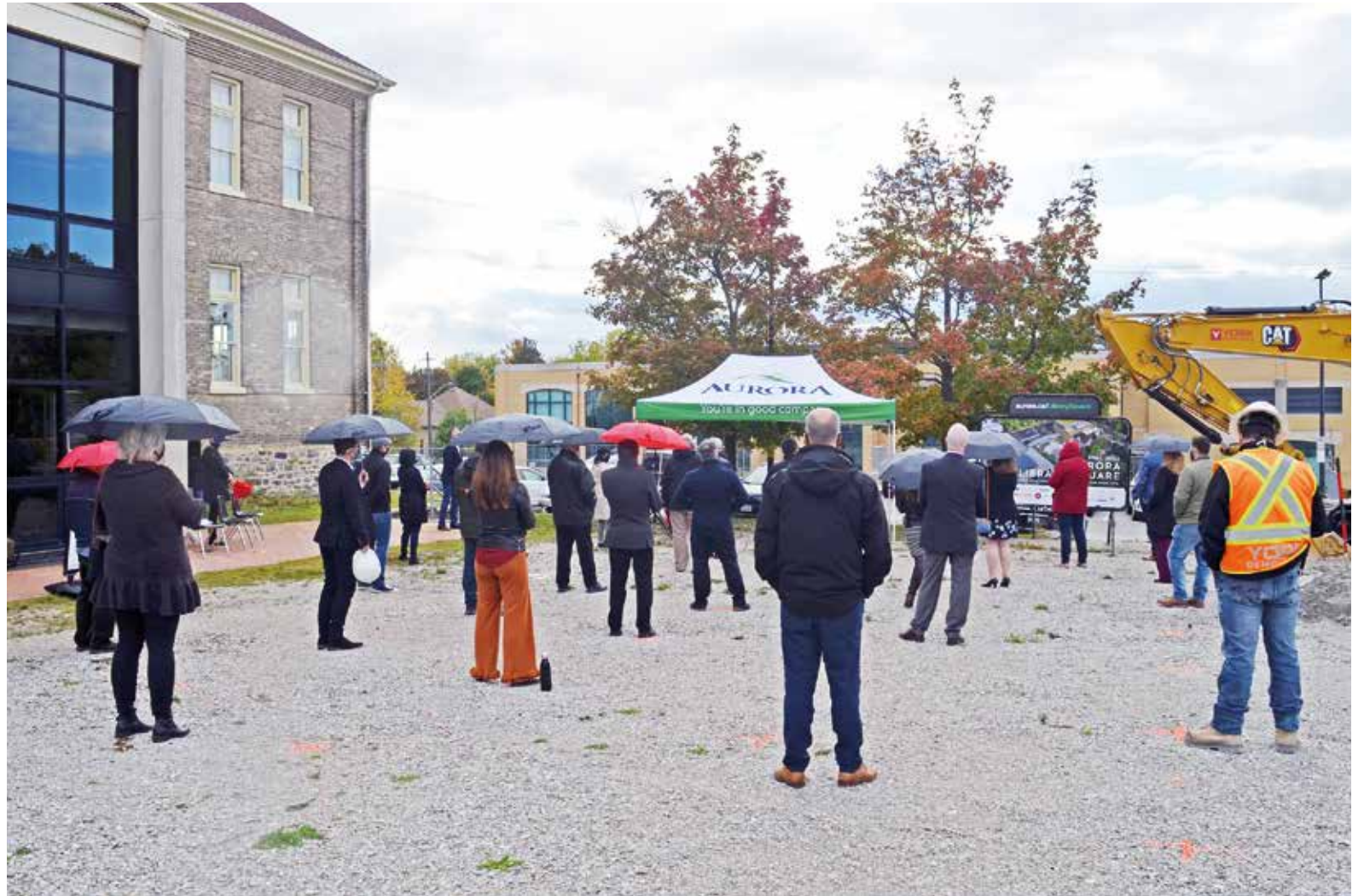
Thursday’s ground-breaking ceremony just behind the historic Church Street School, was a physically-distant affair, with guests standing on places marked out on the gravel in spray paint. Auroran photo by Brock Weir
