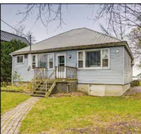
YEAR-ROUND WATERFRONT COTTAGE! $875,000 Charming direct waterfront 4 season cottage. 2 bedrooms, 2 baths, eat-in kitchen and great room with large windows and gorgeous water views. Outdoor oasis boasts large rear deck, boathouse and dock perfect for summer entertaining. Close to town and all amenities, 20 min to Hwy 404!
