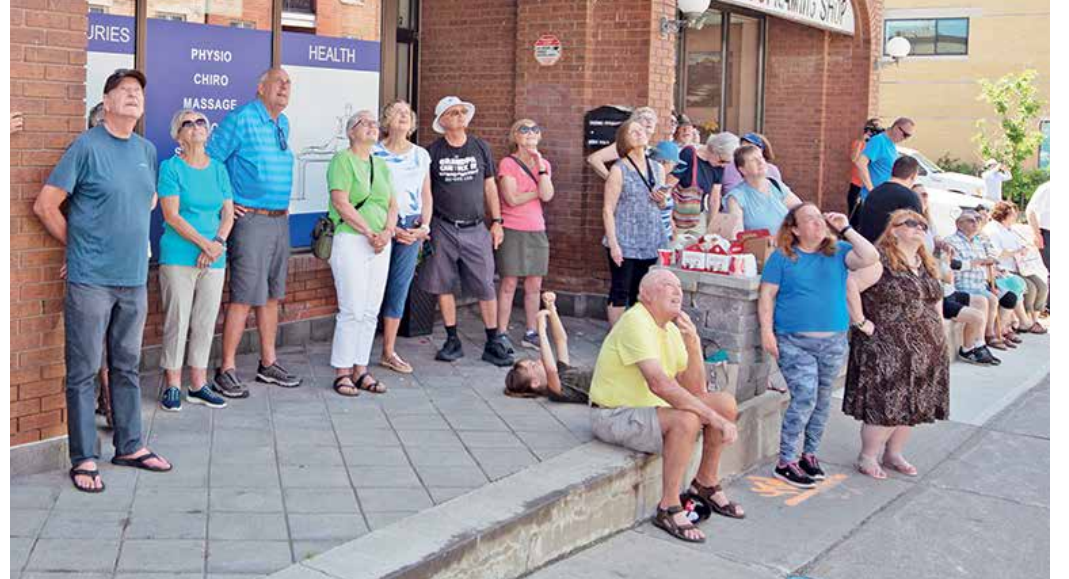
The new home of the Aurora United Church, which was destroyed by fire in April 2014, is continuing to take shape at its historic and spiritual location at Yonge and Tyler Streets. On Thursday, the frame for the south steeple was gently lifted into place as parishioners and community members gathered on Yonge Street's east side to watch the spectacle unfold. Auroran photos by Glenn Rodger
